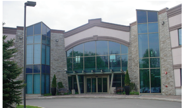
Figure 9: Existing low-rise office building.
